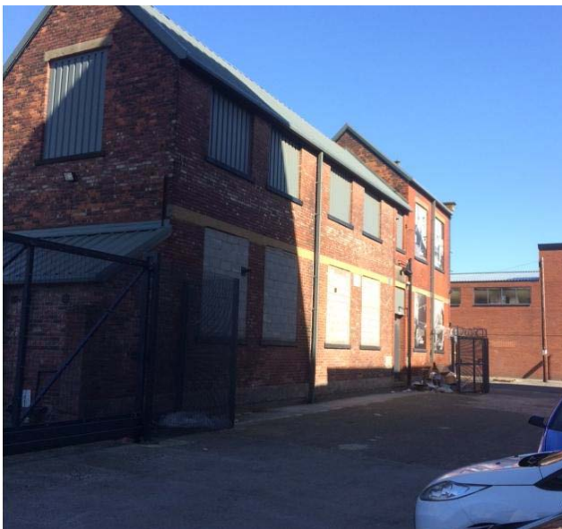
Side view of existing building and the access road – Torah St
